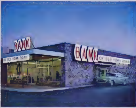
PLEXIGLAS letters and modular background panels at Bank of Old York Road, Abington, Pa. Architects: Haag & Ehrenkrantz
