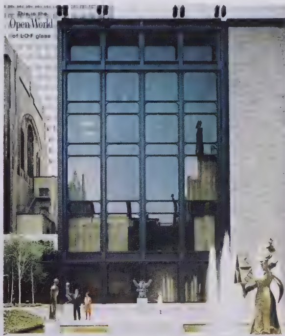
In the new gallery wing of New York's Museum of Modern Art, 3 1/2-inch, heavy-duty Pyralid-O-Bronze® plate glass floods the interior with daylight, yet reduces glare and sun heat. Architects: Philip G. Johnson Associates.
